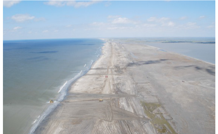
This photo shows the island after construction but before establishment of native beach, dune, and marsh vegetation.
