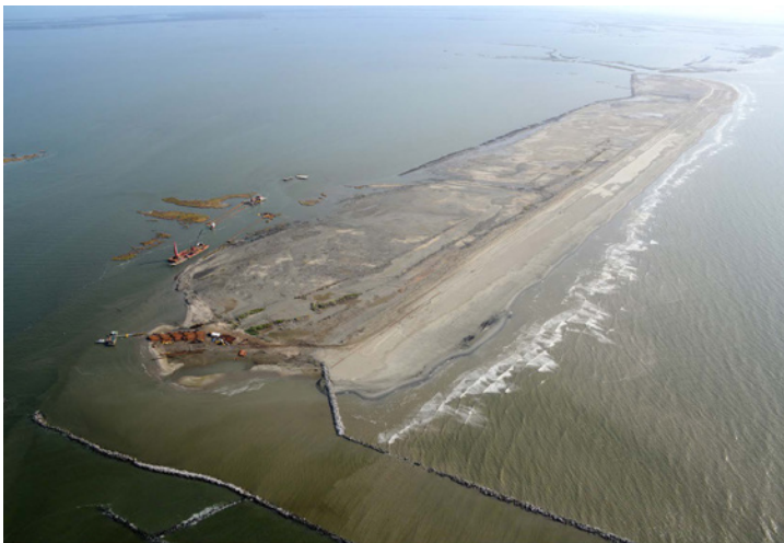
Pelican Island after completion of major construction activities. Large equipment in the lower left of the photo provide a sense of the scale of the project.
