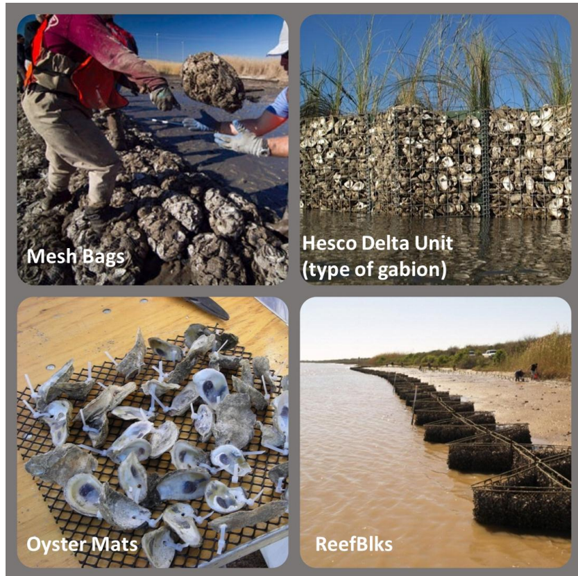
Figure 5. Contained Cultch Designs
