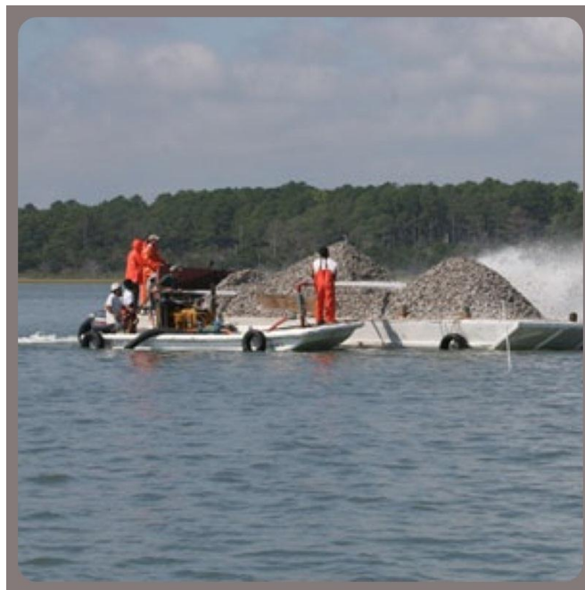
Figure 4. High-Relief Planted Cultch Deployment
