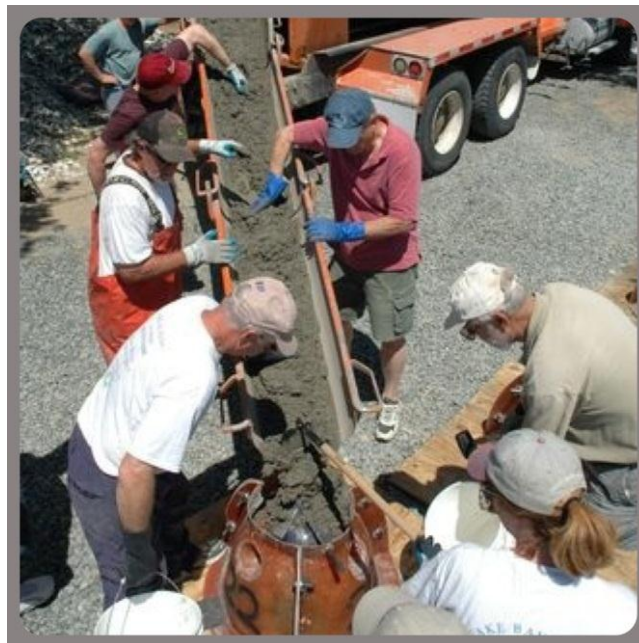
Figure 12. Reef Ball Molds Being Filled on Site
